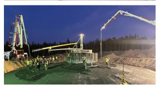
Photos: Project laydown area, pad foundation preparation and pour
