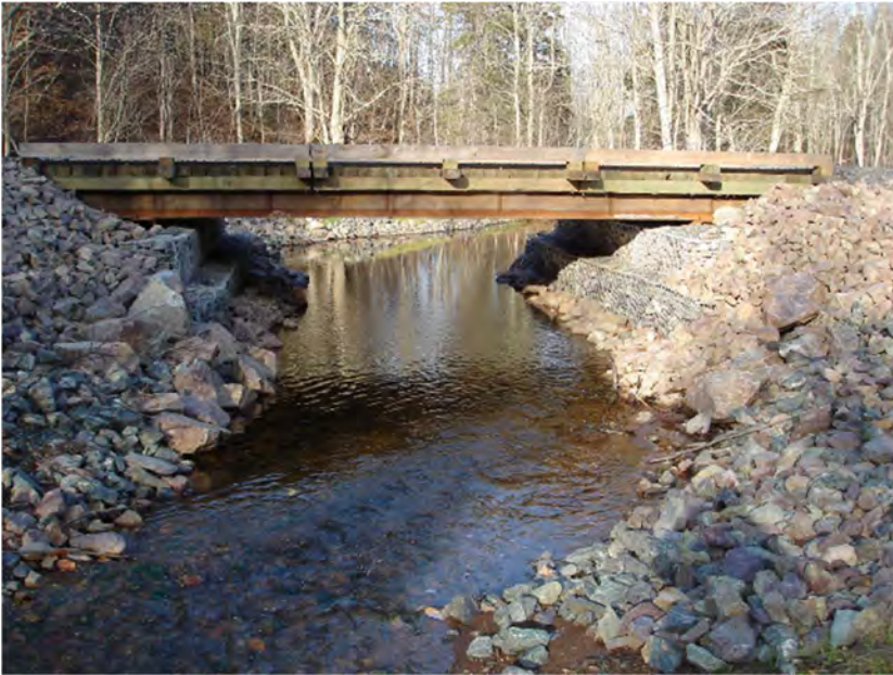
New bridge installation, Paul MacDonald, PHP
